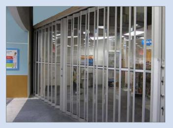
Side Folding Grilles may have curved top tracks for open pharmacy configurations and the curtain stack is often hidden in a side pocket.
