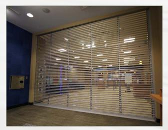
LX6 uses standard housing motors up to 140 sq. ft. Large shutter shown above uses an external motor mounted above the finished ceiling.
