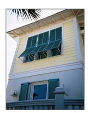
Adjustable arm to control privacy, shading, and for interior operation.
