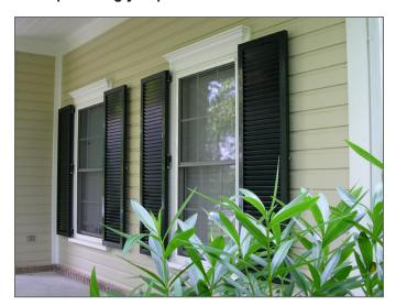
Roll-a-way Colonial Shutters are impact rated. Made from reinforced aluminum, these shutters pass the large and small missile impact test and meet HVHZ's stringent requirements.
