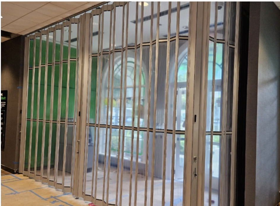
In-process installation of QMi Q-Clear Side-Folding Grille shipped with protective film over poly panels.
