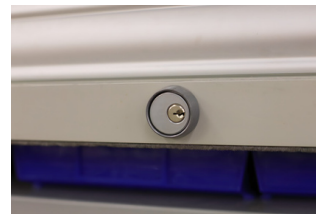
Base Slat Cylinder Lock
