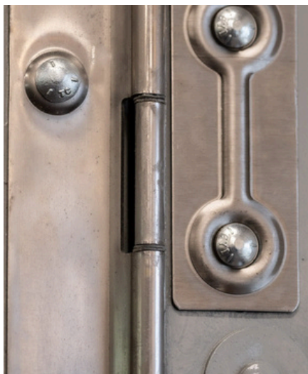
Continuous hinge and interlocking astragal protect against pry attacks.
