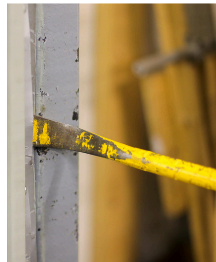
Continuous hinge and interlocking astragal protect against pry attacks.
