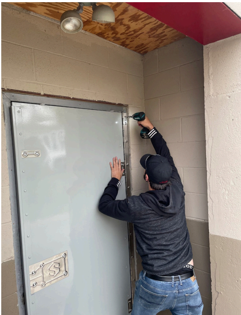
An expert QMi installer secures the continuous hinge on the QMi replacement door.
