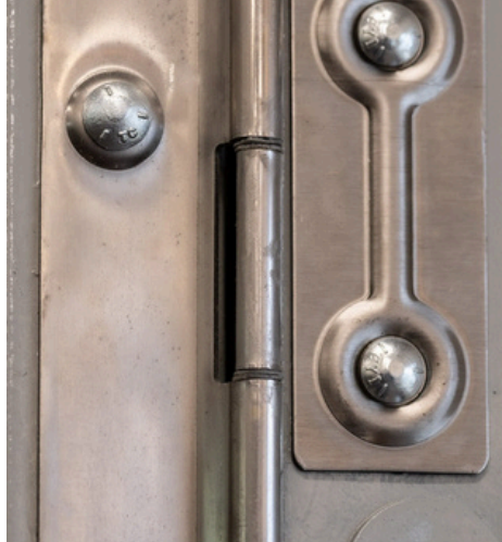
Continuous hinge and interlocking astragal protect against pry attacks.
