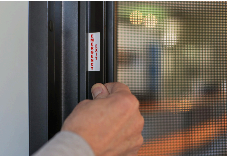
Egress screens are easily opened using the panic bar shown here.
