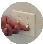
Wall Switch (Motor)
